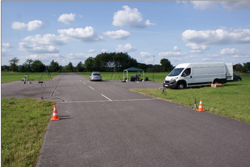
Figure 21. View of test section on ISO2
