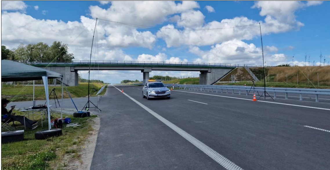
Figure 11. Measurement location at Szemud (Poland)
