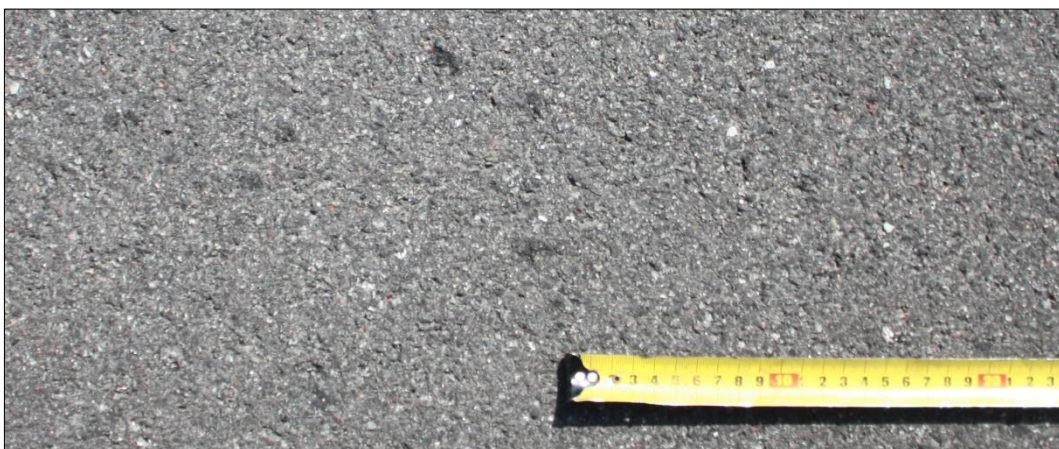
Figure 6. Ma11 road surface
