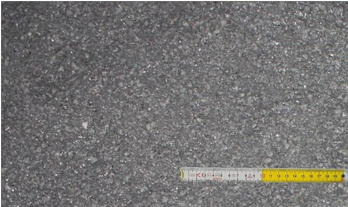
Figure 10. SMA11 road surface
