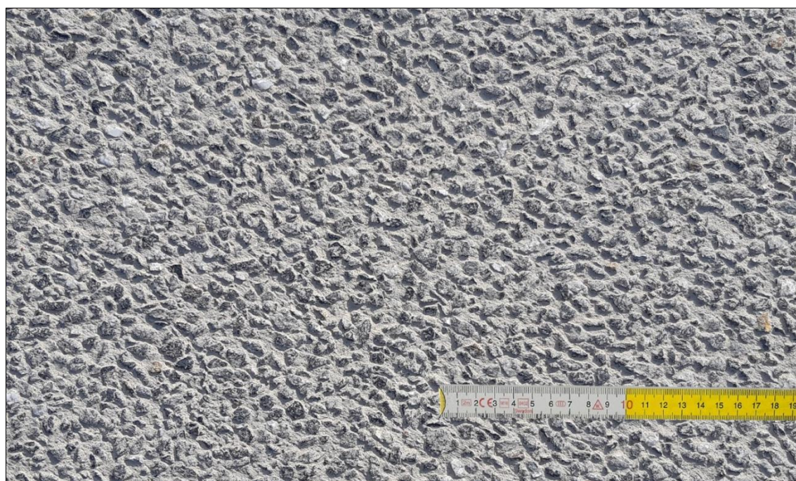
Figure 12. EACC road surface
