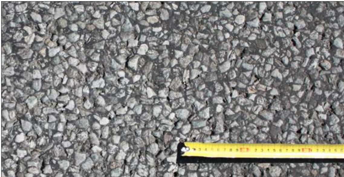
Figure 6. SMA16 road surface
